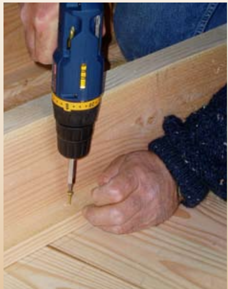
The T-beams are screwed to the bottom.
