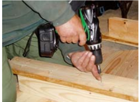
The T-beams are screwed together.
