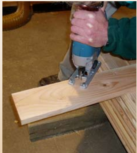
The fixing boards are cut into length along the carved line.
