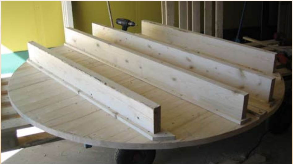
The fixing boards and the bottom joists are screwed together into T-beams, which then are screwed to the bottom. The ends touch the 20 mm line.
